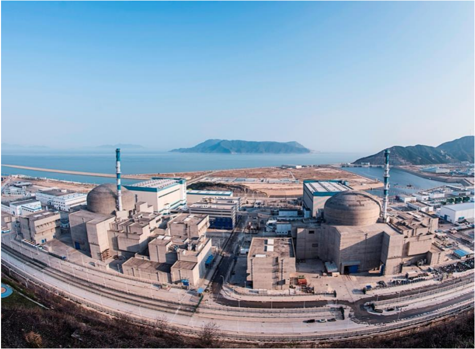
EPR-1750 reactors at Taishan Nuclear Power Plant, China
