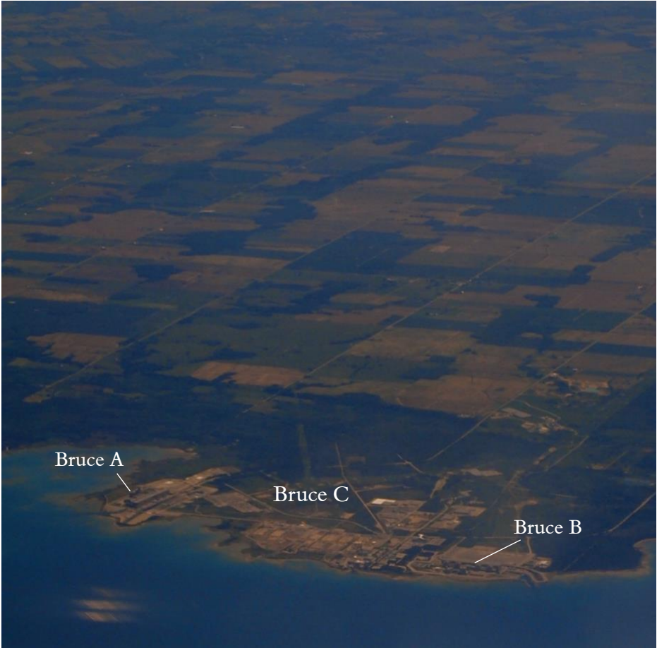
Aerial view of Bruce Nuclear Generating Station, Bruce County, Ontario. The site currently provides around 30% of Ontario's electricity. Bruce C's approximate future location is labeled
